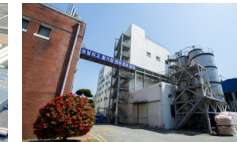
Jeonju EP Plant
