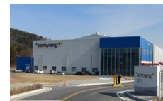
Daejeon EP Plant
