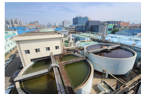
Wastewater treatment facility at Incheon Plant 1
